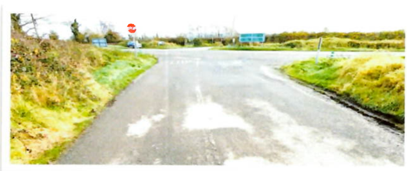
Figure 2.2 – Depleted Stop Road Markings on L-5040 Approach to the N52
